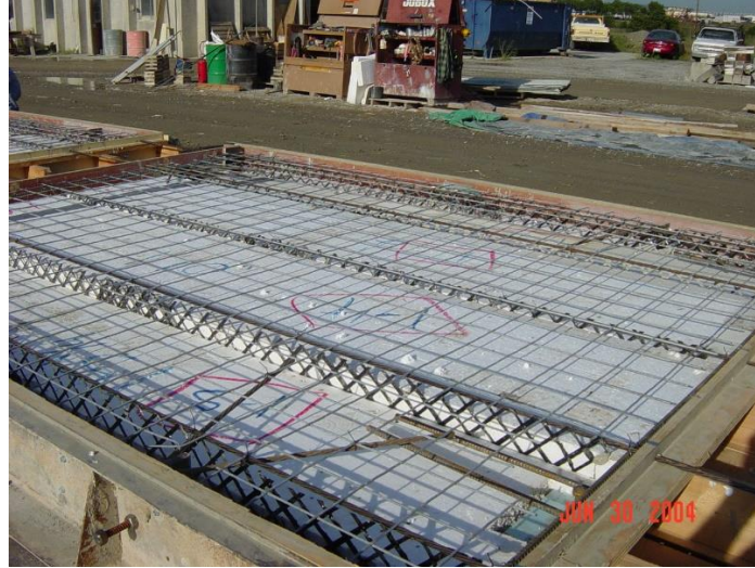
Figure 2.2 Typical sandwich panel production prior to placing top concrete wythe
