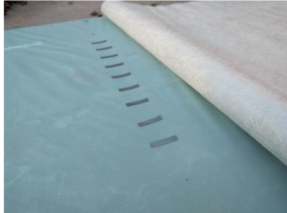
Figure 3.5 Attaching solar cells and laying down the glass fiber CSM
