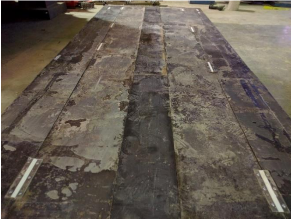
Figure 3.4 Formwork with four rubber connection at each side
